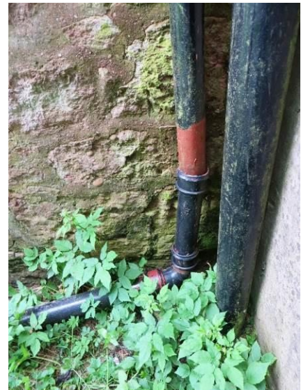
Figure 15: cast iron gutter in need of painting and is liable to choking from pine needles from neighbouring trees. Render and timber windows in poor repair; (below) hopper at junction of Hall and Nave also liable to choking and the downpipe is out of alignment.
