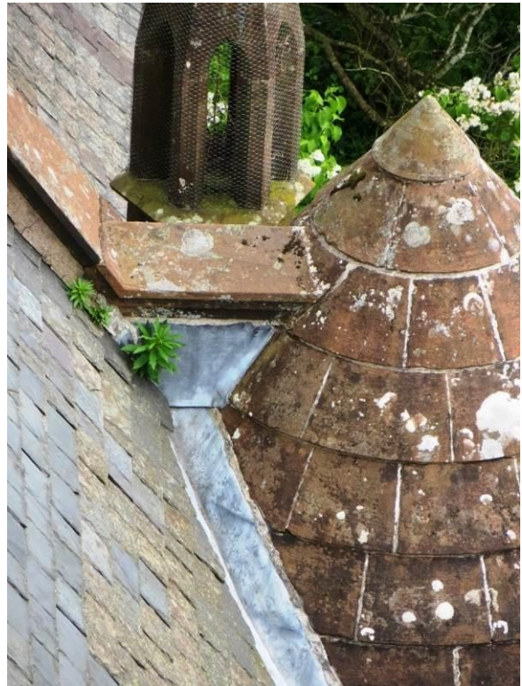
Figure 7: Effects of water penetration on the south wall behind the organ and externally the complex junction of Nave / Tower /Porch; (below) effects of water penetration at the south corner of the east gable possibly a failure of the lead flashing and / or mortar skew fillet below the cope.
