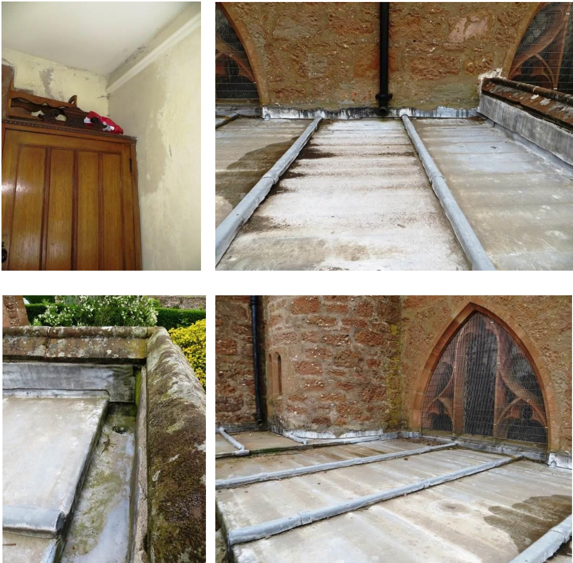
Figure 12: The Vestry has signs of water penetration and mould growth in a number of areas thought to be caused by multiple failures in the ageing lead roof.
