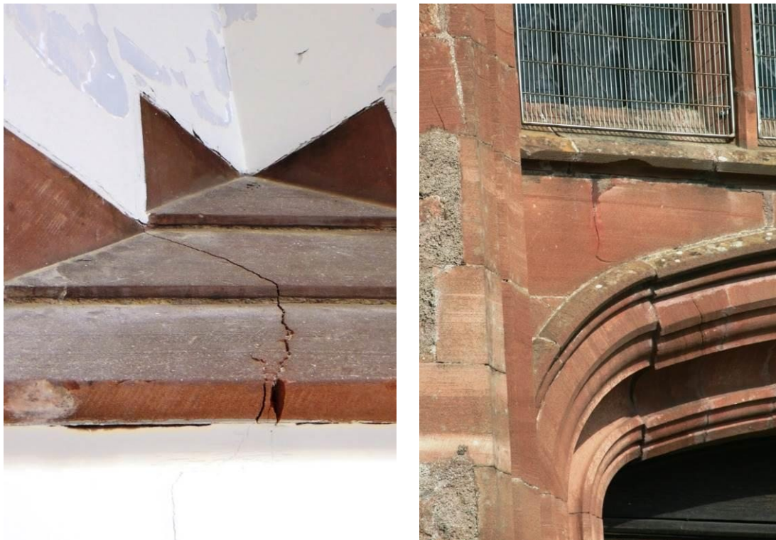
Figure 15: Movement cracks through stonework in the West Tower: over internal access door to stair (left) and above west entrance.
