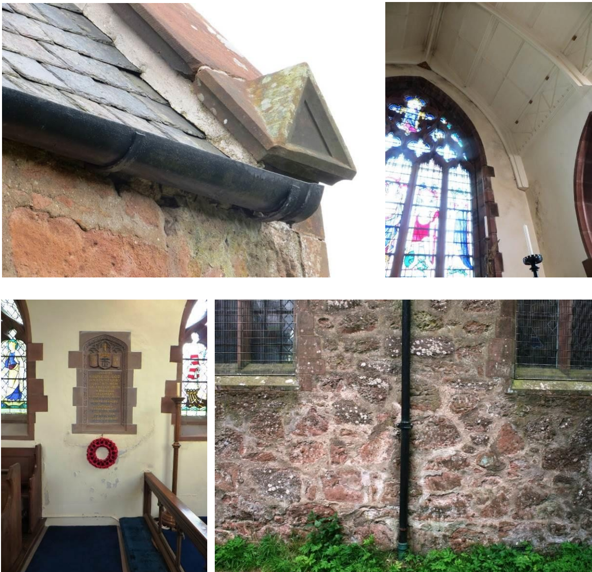
Figure 13: The roof junction is only protected by a mortar skew fillet which has lifted off the slate; the east gable of the Chancel shows signs of water ingress at high level and extending down the wall; (below) signs of water penetration and flaking paint finishes below the war memorial, may be historic from defective rainwater downpipe; externally masonry shows signs of erosion around this pipe.
