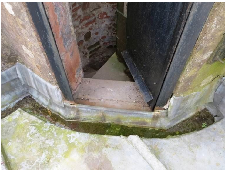
Figure 5: (From top) parapet masonry in poor condition; previous cracking on W elev; plant growth in open joints; cracked cope; water ponding at stair door; water ingress in belfry below stair door.
