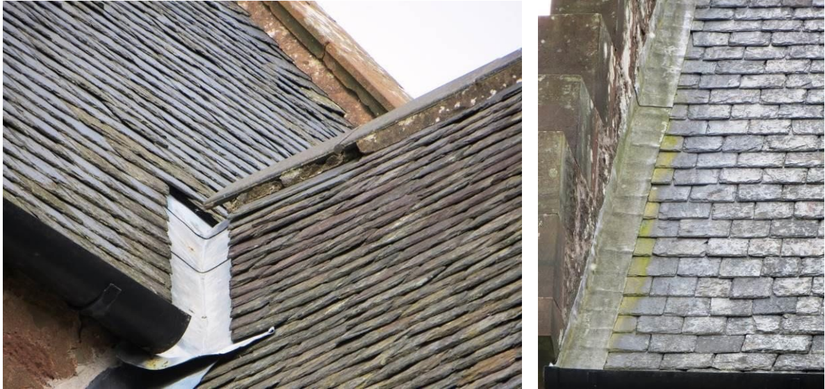
Figure 10: Damaged bedding mortar below clay ridge tiles; ageing over flashing at the roof abutment with the gable.
