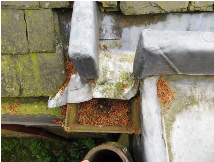
Figure 15: cast iron gutter in need of painting and is liable to choking from pine needles from neighbouring trees. Render and timber windows in poor repair; (below) hopper at junction of Hall and Nave also liable to choking and the downpipe is out of alignment.
