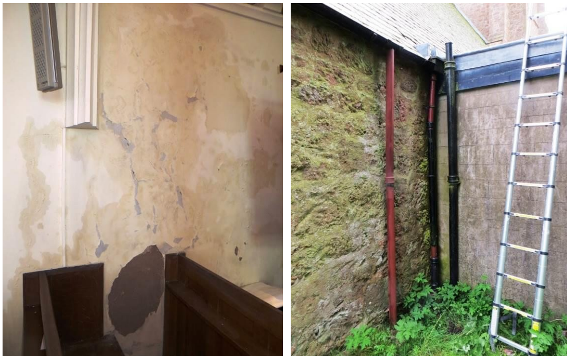
Figure 8: Effects of water penetration above and around the window in the north aisle. (below) damaged plasterwork in the north aisle coincides with downpipes and hopper at hall junction.
