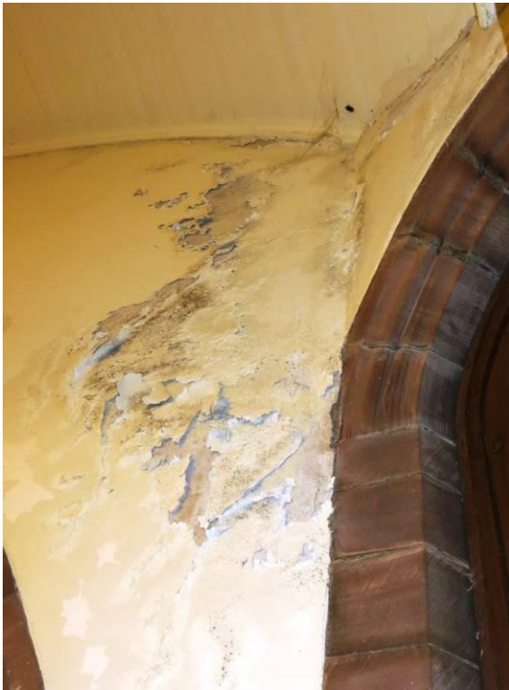
Figure 7: Effects of water penetration on the south wall behind the organ and externally the complex junction of Nave / Tower /Porch; (below) effects of water penetration at the south corner of the east gable possibly a failure of the lead flashing and / or mortar skew fillet below the cope.
