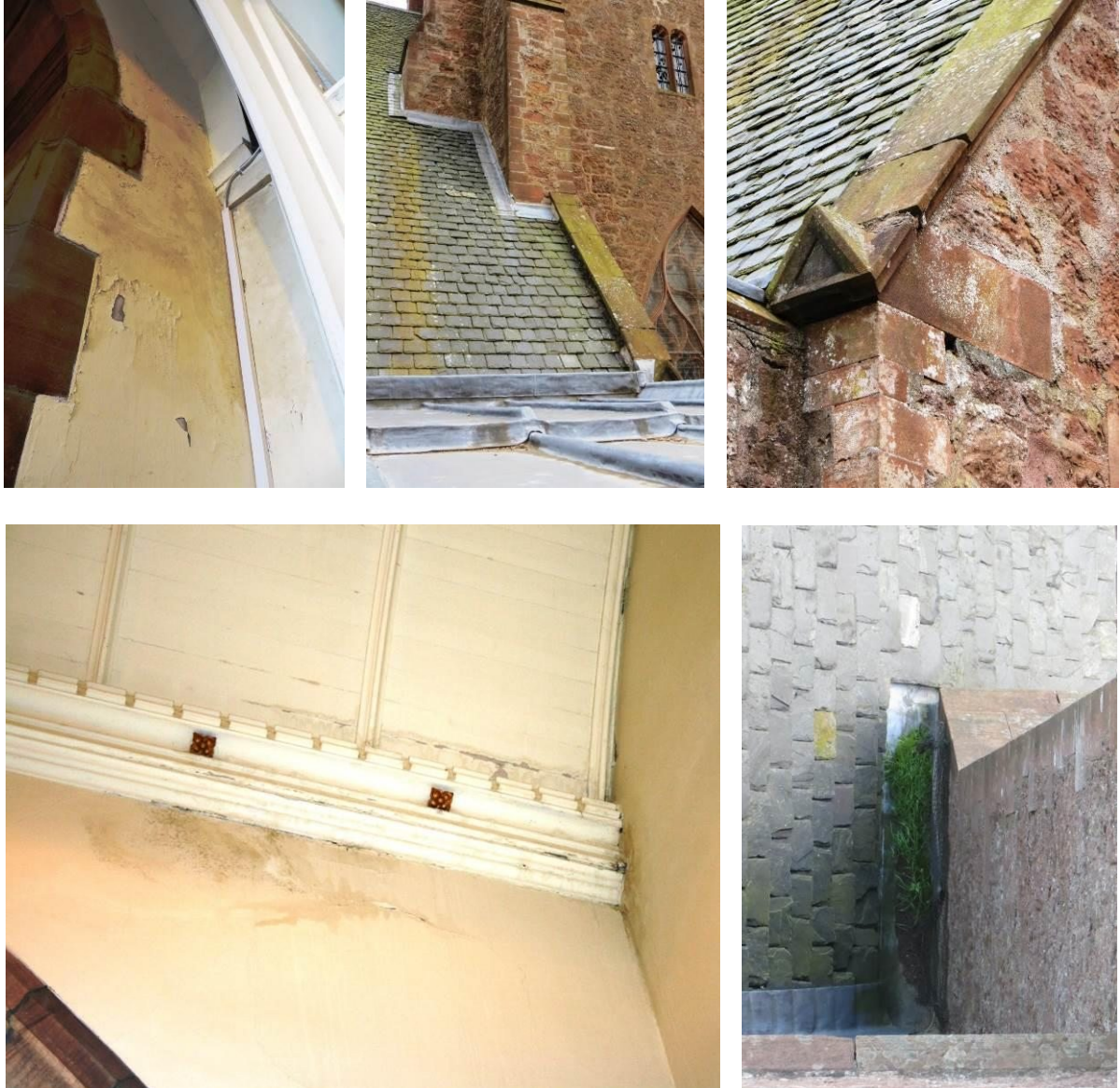
Figure 9: Effects of water penetration on the west wall of the aisle; the roof junction is only protected by a mortar skew fillet and the masonry to the copes and gable wall head is in need of repair. (below) effects of water penetration at eaves level on the south elev; blocked lead gutter behind the buttress.
