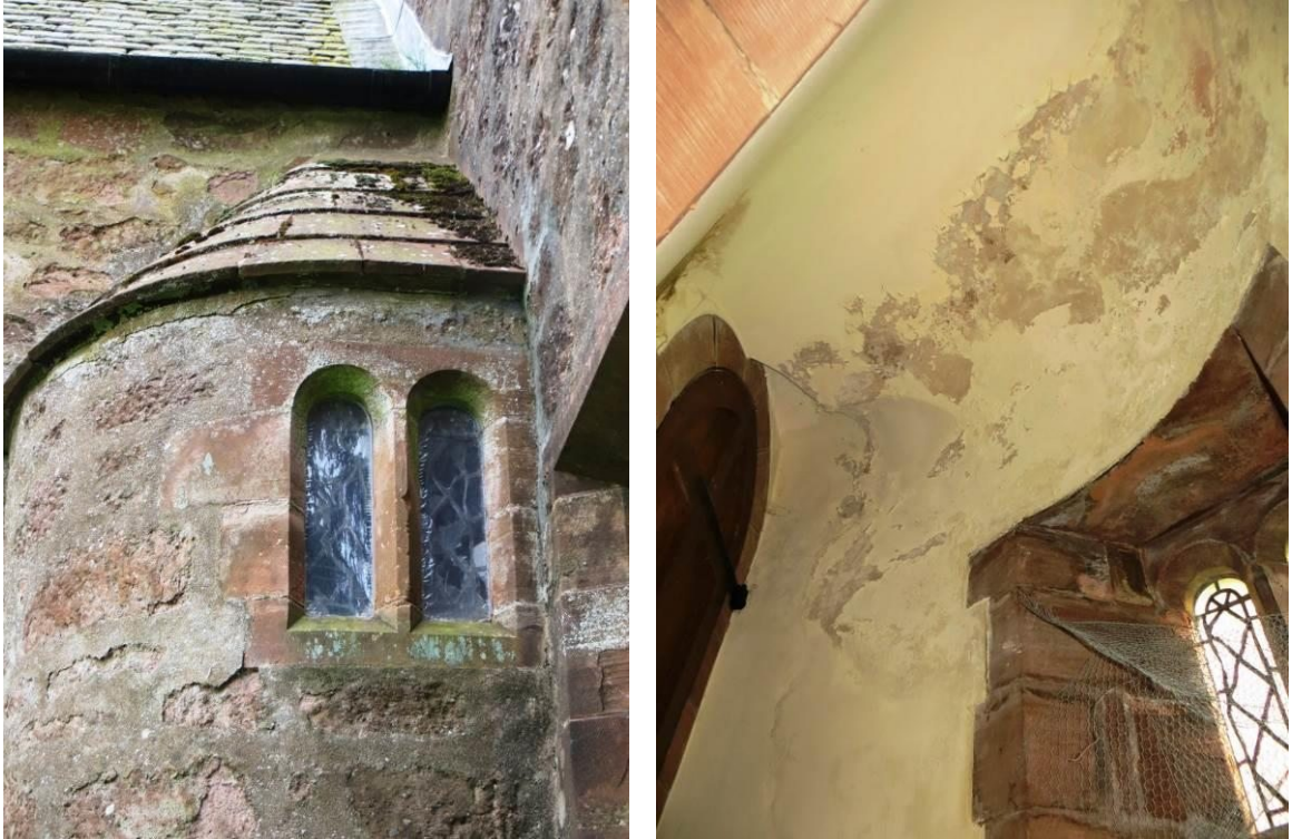
Figure 14: the NE stair tower with stone capped roof and no flashing at junctions with Chancel and east gable wall of Nave; effects of water penetration internally.
