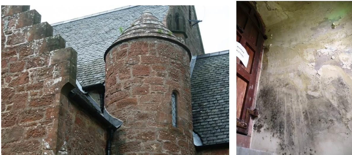
Figure 11: The stone capped SE tower abuts the Nave / Porch and Chancel; water penetration has damaged the internal plaster finishes particularly around the upper door to the Nave.
